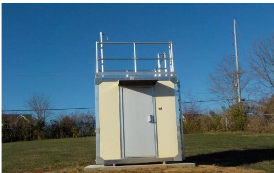
Figure 43: Buckner Air Monitoring Shelter
