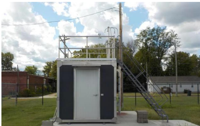
Figure 65: Paducah Transit Air Monitoring Shelter
