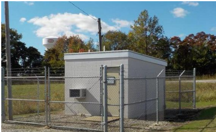
Figure 71: Sebree Air Monitoring Shelter
