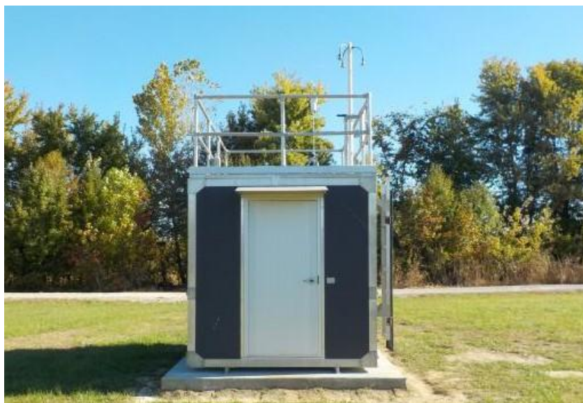
Figure 59: Meadow Lands Air Monitoring Shelter
