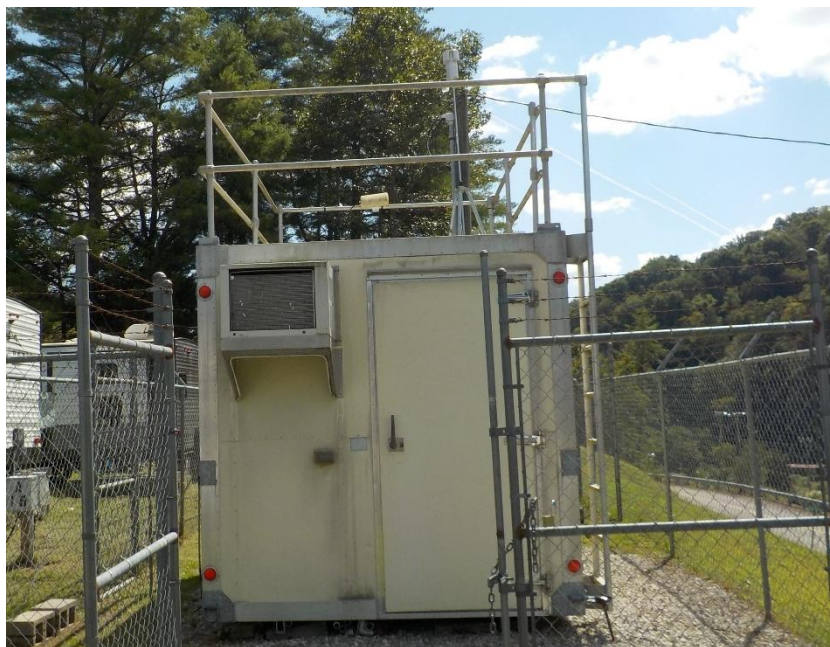
Figure 86: Hazard Air Monitoring Shelter
