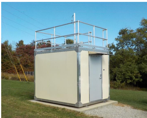
Figure 9: Nature Center Air Monitoring Shelter
