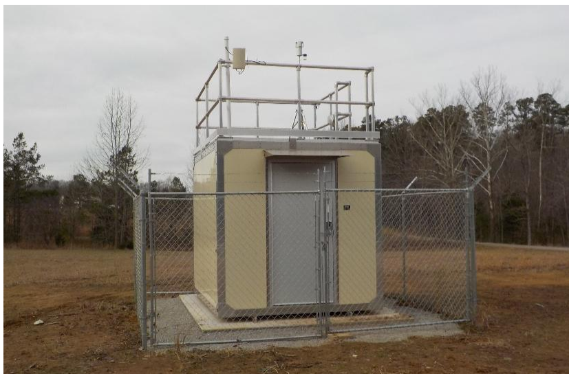
Figure 15: Pennyrile Forest Air Monitoring Shelter
