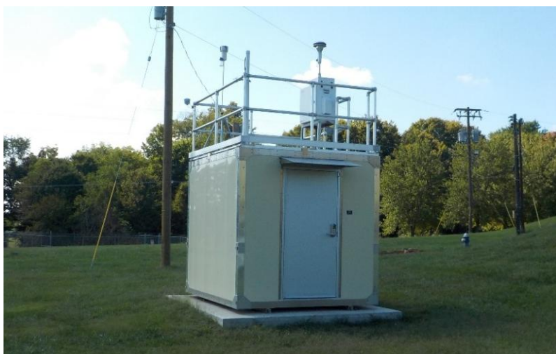
Figure 18: Freeman Lake Air Monitoring Shelter
