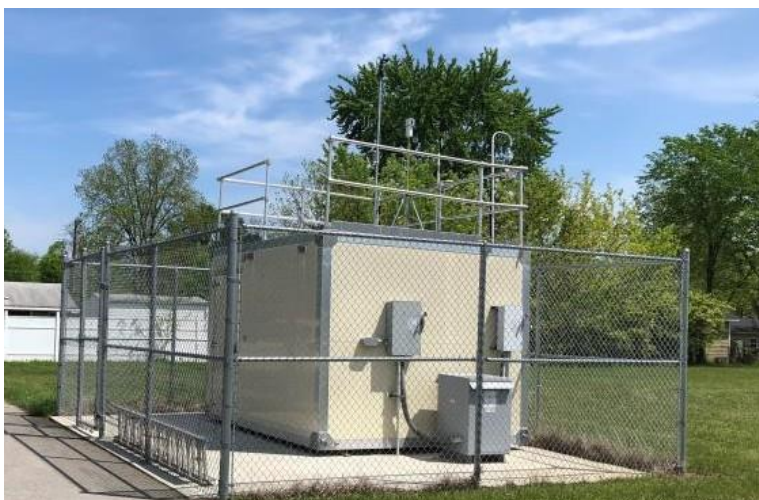
Figure 54: Carrithers Middle School Air Monitoring Shelter
