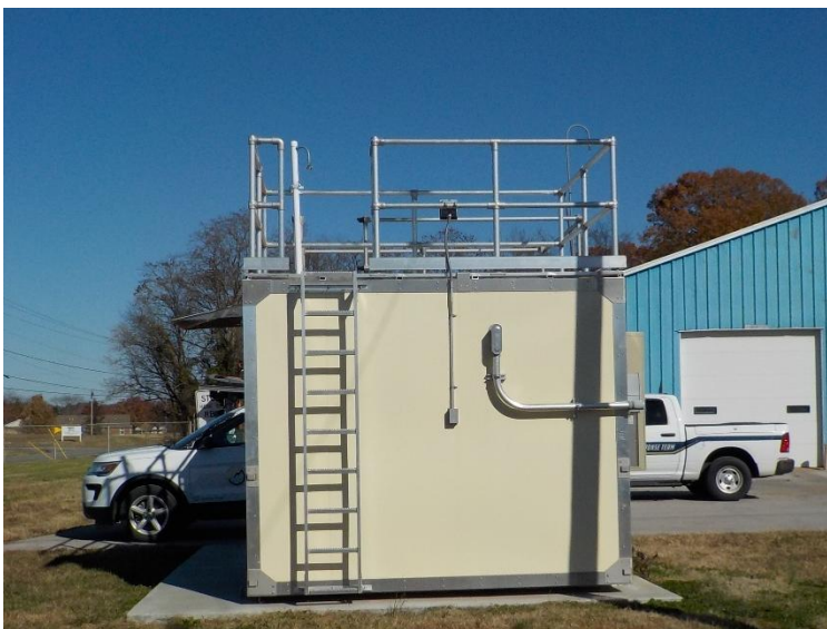
Figure 81: Franklin Air Monitoring Shelter
