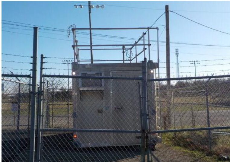
Figure 41: Shepherdsville Air Monitoring Shelter
